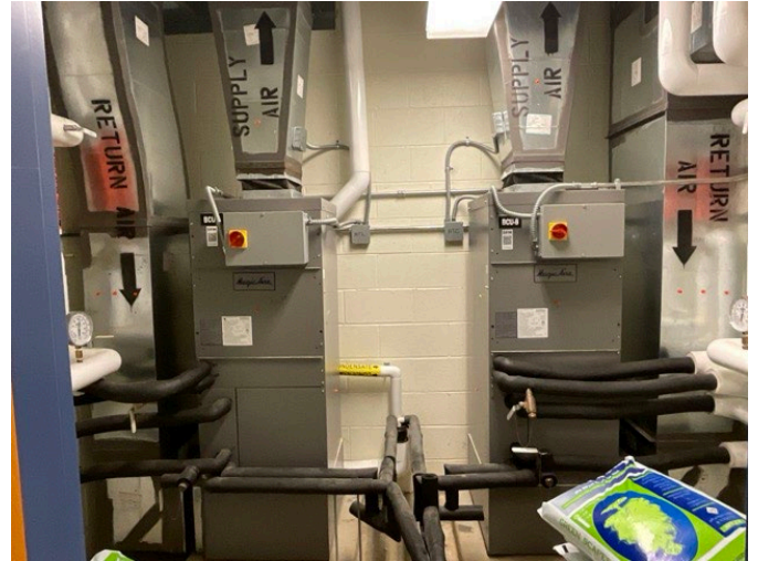
26 - MECHANICAL CLOSET (2ND GRADE WING)
