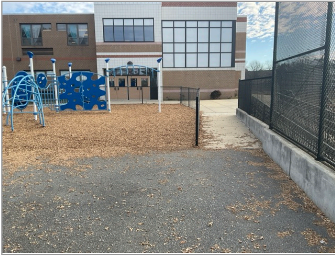
ACCESSIBLE ROUTE TO PLAYGROUND
